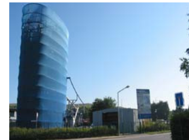
Biomass Gasification: Blue Tower
