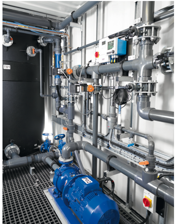
Bioreactor and membrane sidestream pump
